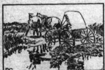
earth roads and should be used after each rain. On a heavy clay or gumbo soil the drag when properly used tends ddle the road surface, keep it free from ruts, dense, smooth and hard, thus securing the best surface drain
